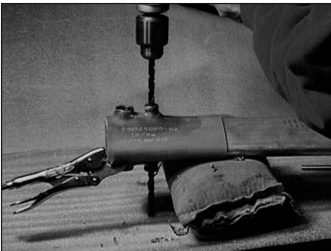
Figure 73: Drilling the Inboard Holes
