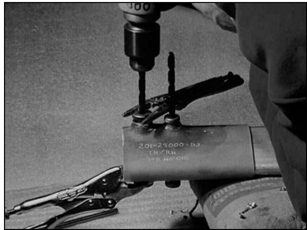
Figure 74: Drilling the Outboard Holes
